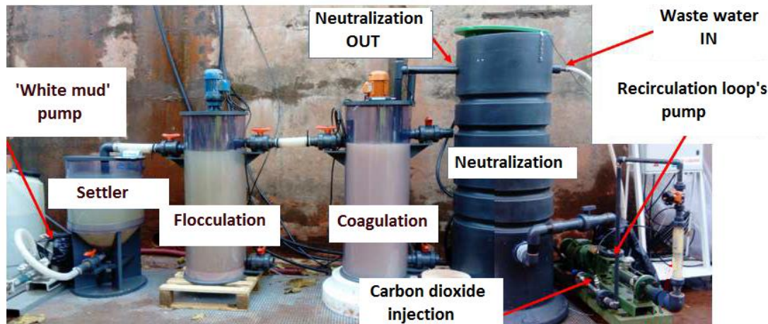
Figure 5. Carbon dioxide neutralization pilot plant.
